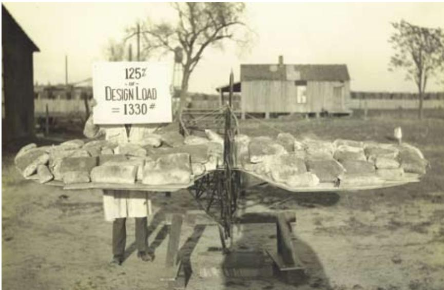
**In this factory photograph by R.D. Wolff a horizontal stabilizer of a model 3C3 is being load tested. Holding the sign is none other than designer Albert Vollmecke. Albert always designed with a great margin of safety in all his ships.**
